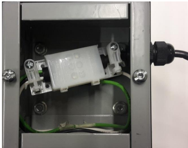
Fig. 43 Completed electrical connections to the projector 74-00013-01
